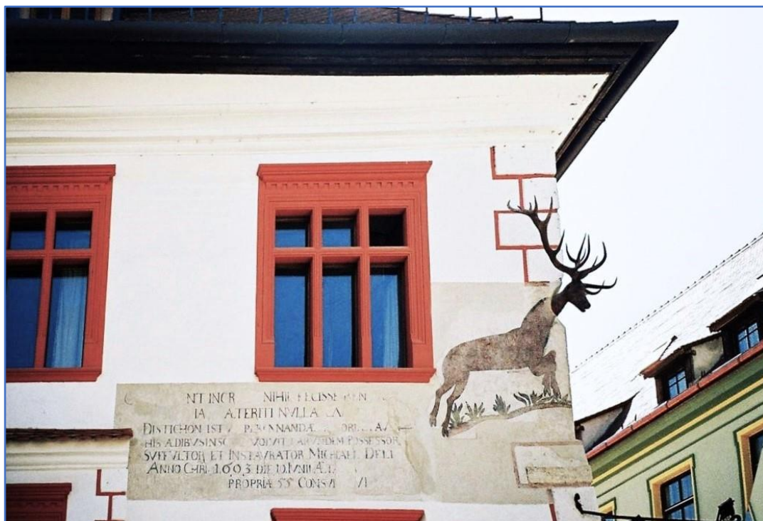
Fig. 2. – The Stag House, the inscription painted in 1693 on the façade, 2006.
