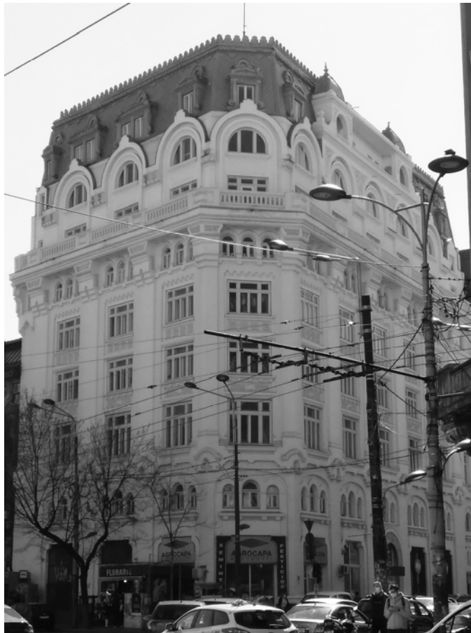
Fig. 7 – Societatea Comunală de Locuințe Ieftine Building, 1924, collaboration with architect Jean Pompilian, Bucharest.
